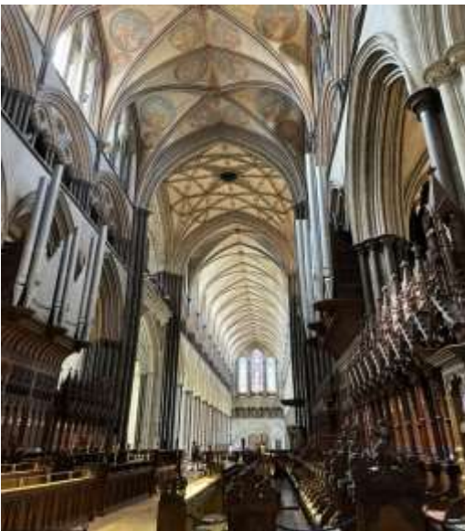
The Nave looking West
